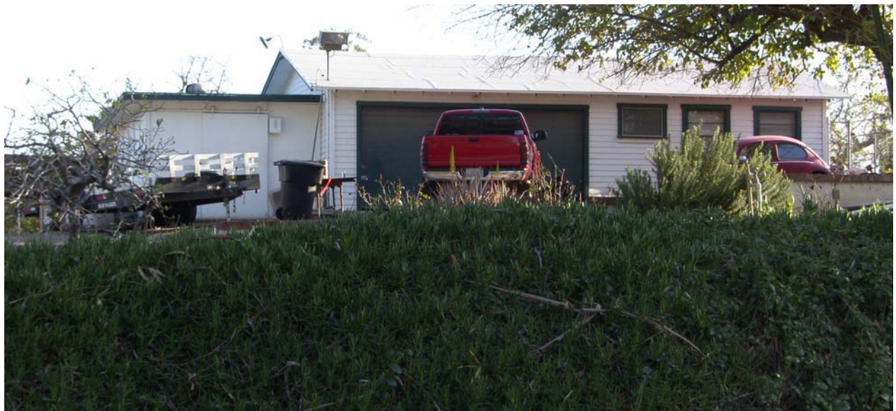
Photo 16 - Garage Looking South
