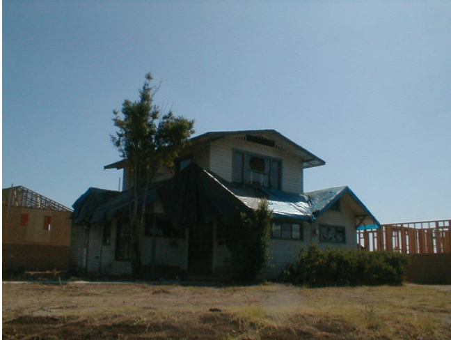
Photo: Corner facing facade (taken by GPA, July, 2005)
